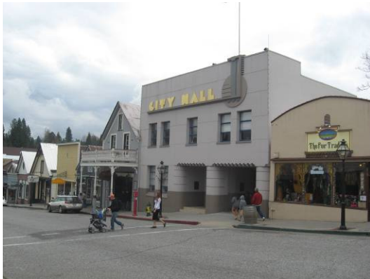
The uncontrolled marked crosswalk in front of City Hall has standard striping
