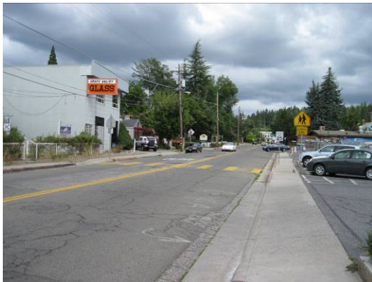
The uncontrolled marked crosswalk in front of Hennessy Elementary School requires a crossing guard for safe passage by school children
