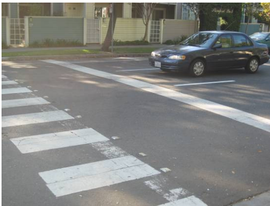
Advanced stop bars are placed in crosswalks; they keep vehicles from encroaching into the crosswalk when stopped at a red indication
