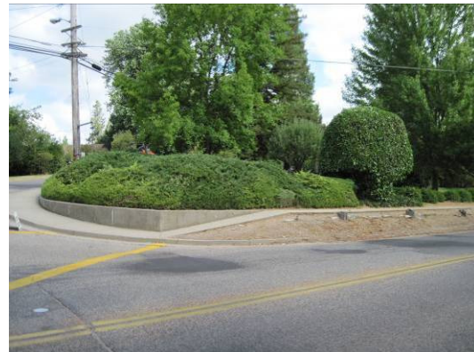
Lowering the sidewalk to street level on Sacramento Street would improve accessibility
