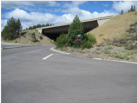
Sidewalks are missing on key segments of Donner Pass Road, including under the I-80 interchange
